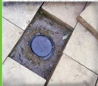
Installation under pavers
